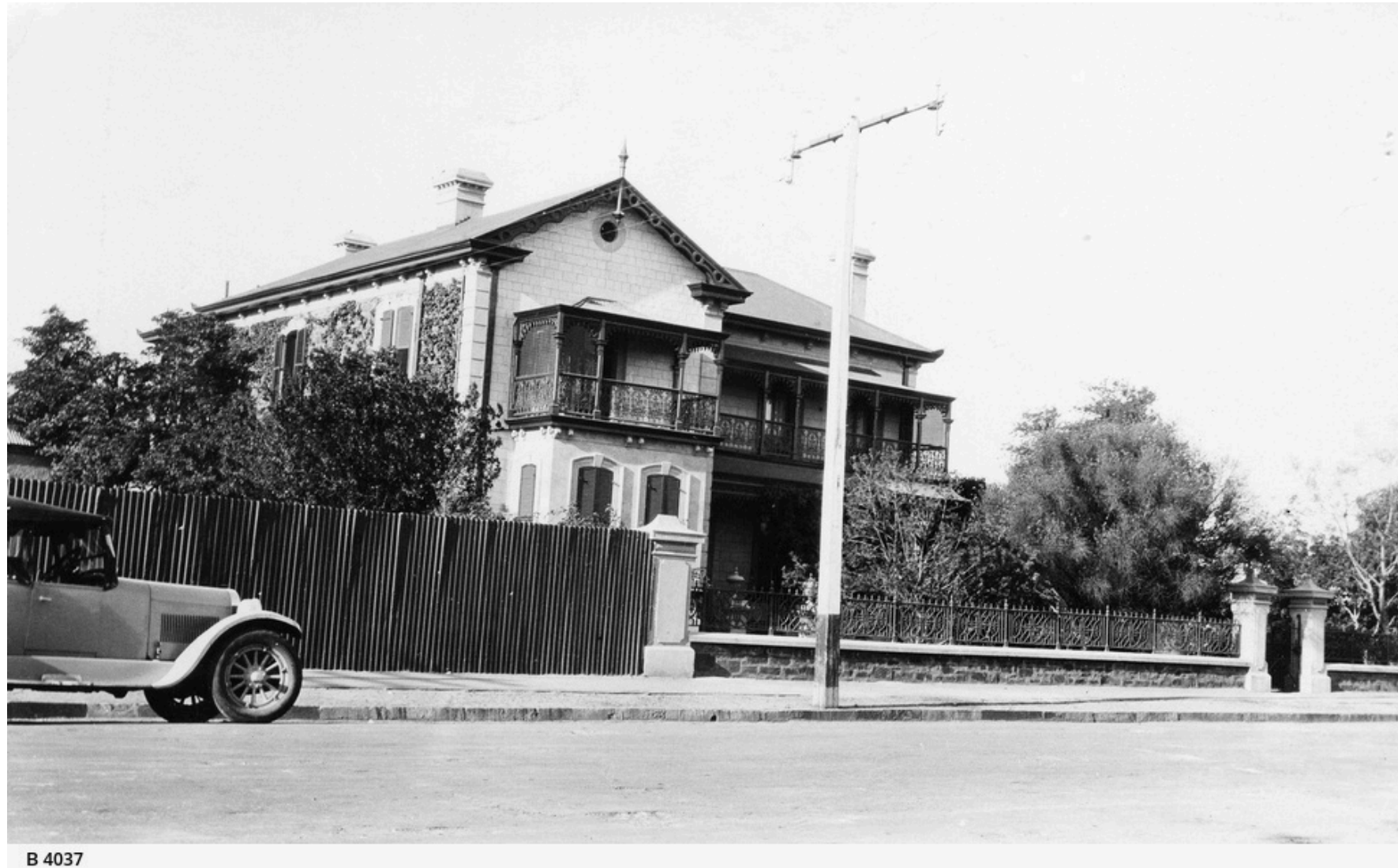
Wheaton House as a private residence
