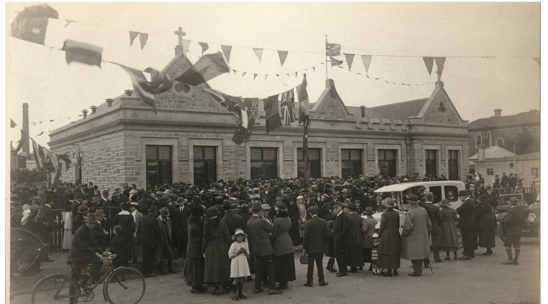
The opening of Nicholls Building in 1921.
