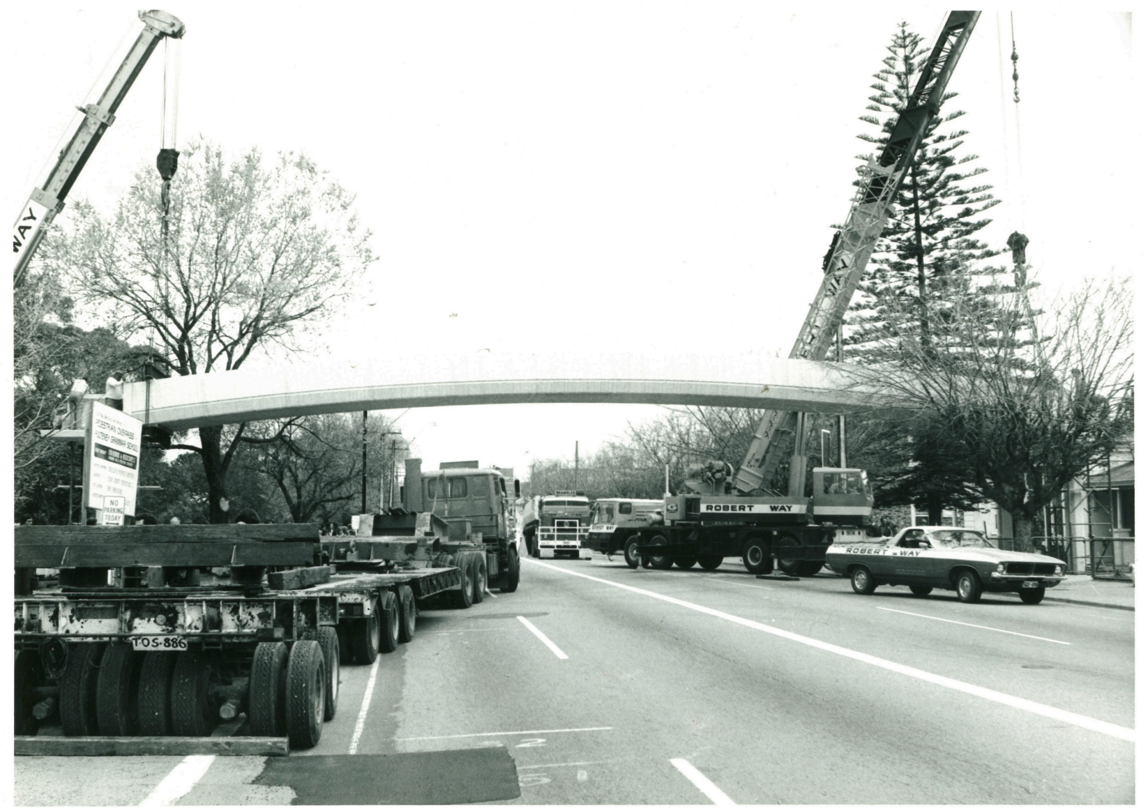
The overpass being put into place.
